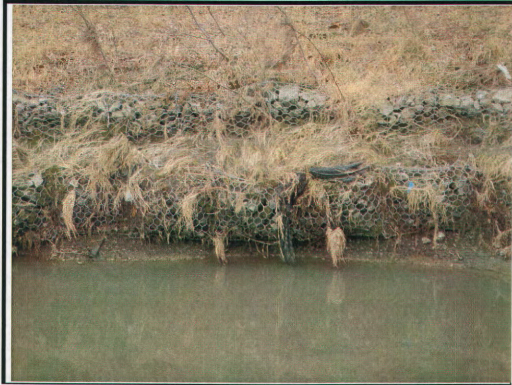
PHOTO NUMBER 3 View showing bank exposed below gabions (upstream of slide)
